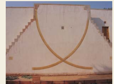
The East facing wall of the Dakshinottara Bhatti
